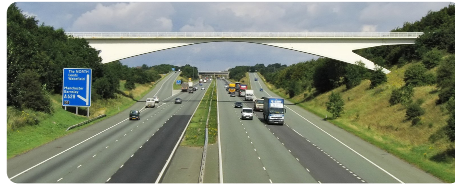
M1 motorway in Yorkshire
